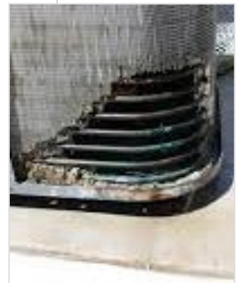
Effects of corrosion on a typical air side Copper-Aluminium exchanger, installed on a unit located in a urban ambient, with high level of atmospheric pollution.
